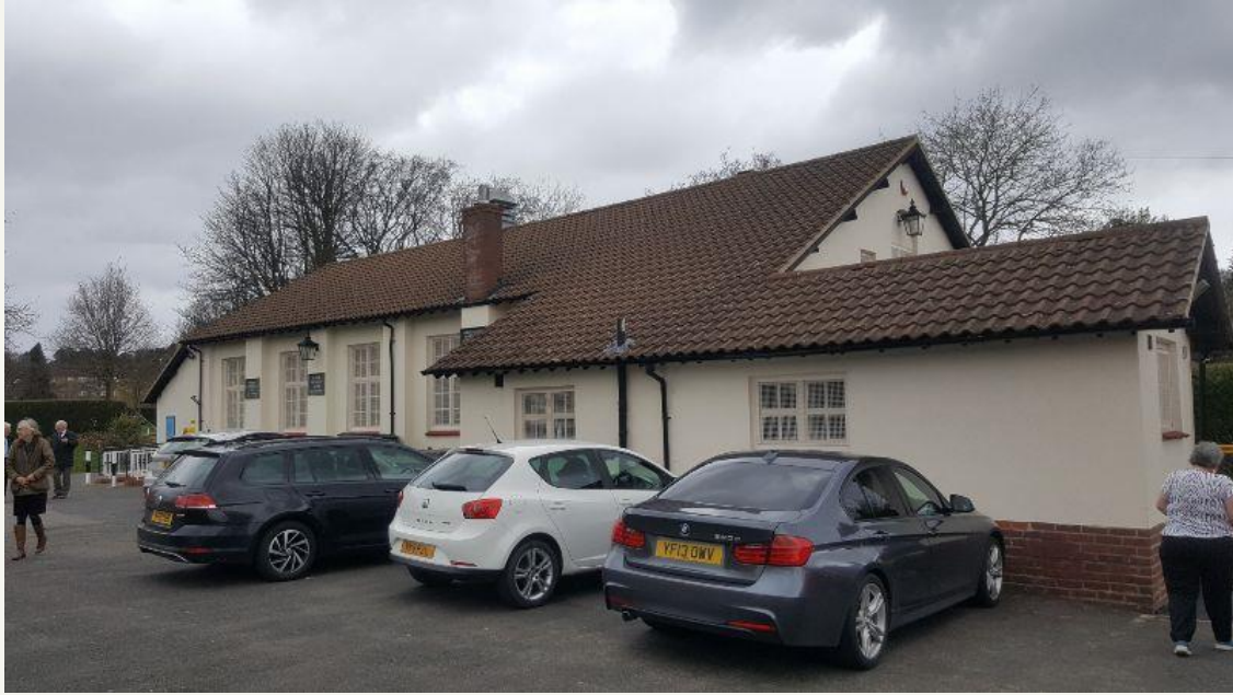
Weoley Hill Village Hall is used by badminton and tennis clubs, and was recently expanded.
