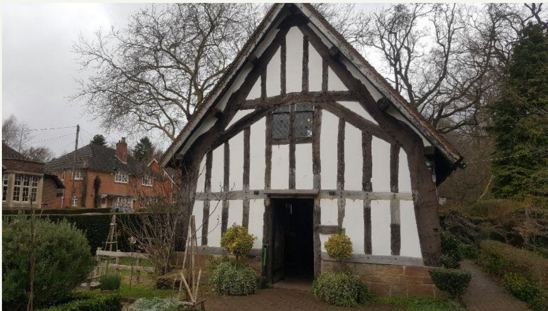
Minworth Greaves is the oldest building on the Bournville Estate. It's a timber cruck framed, Grade II listed building, thought to date from the 14th-century or earlier, possibly as early as 1250. It was originally built in Minworth, near Sutton Coldfield to the north of Birmingham. After falling into extreme disrepair, it was purchased by George Cadbury and re-built by Laurence Cadbury in 1932 in the grounds of Selly Manor.
