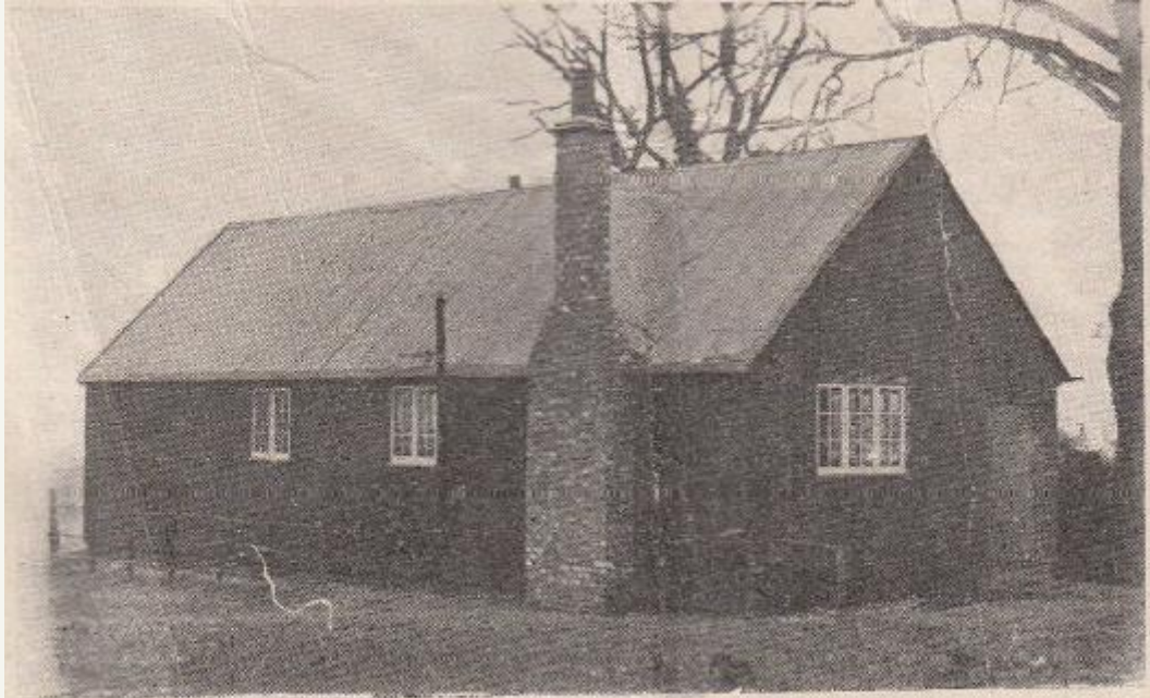
TEMPORARY VILLAGE HALL Built by workers in their spare time. Opened 11th October, 1919
