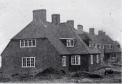
These are the first group of cottages to be inhabited, known as Group A, on Green West Road. Building commenced in March '19 and was completed in Dec '19
