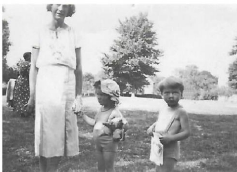
On the village green, with Des, Emmy and Ricky; and watching the steam roller, mending the road.
