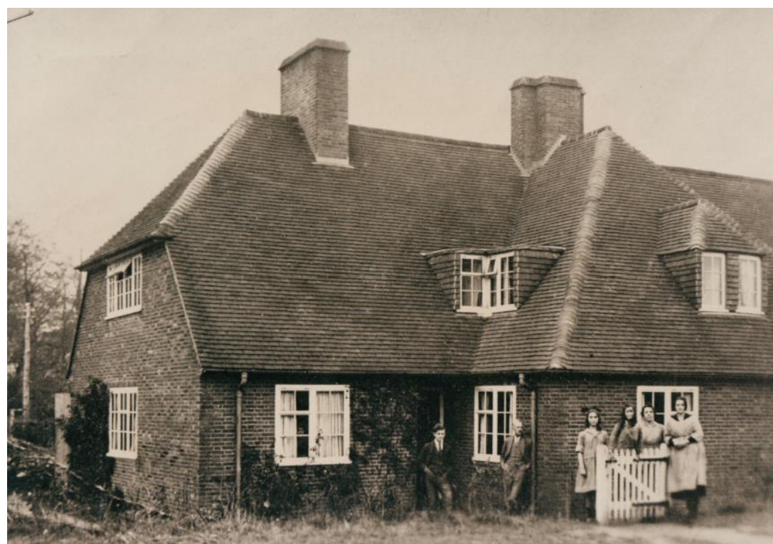
Above Right: The Homestead, Green West Road
